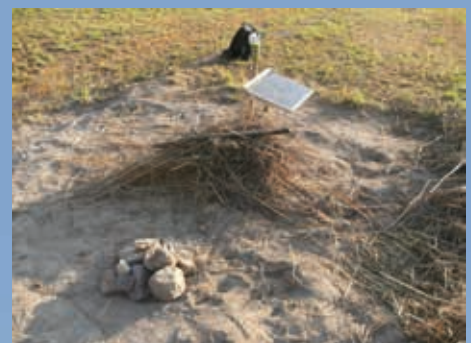
Typical finished site for seismometer deployment. The rocks show the location of the seismometer, the twigs show the battery bucket location and the solar panel and GPS sensor stay above ground.
