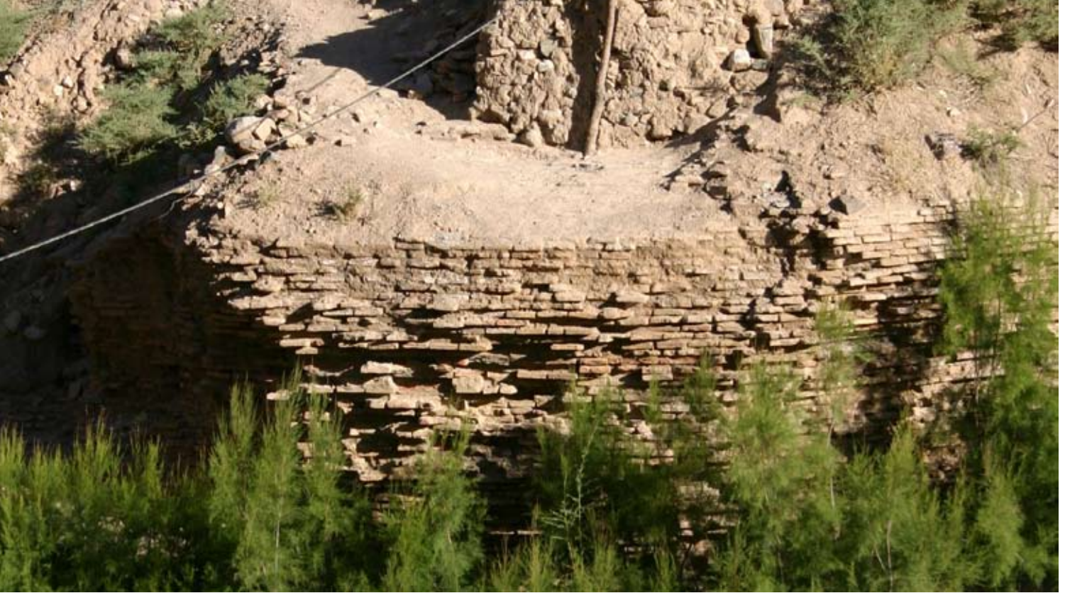
The brick foundations of the Ghurid bridge which once spanned the Hari Rud at Jam.
