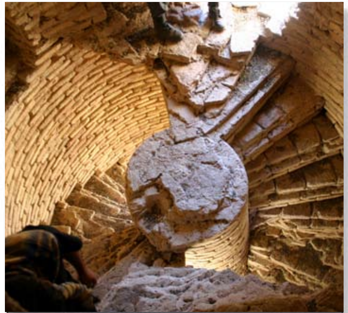
The interior of the minaret.
