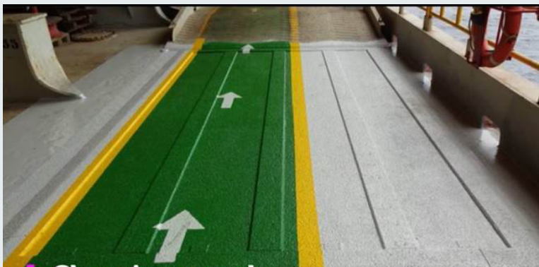
Figure 5: Cold Pad applied to repair the corroded deck (Courtesy of Cold Pad)
