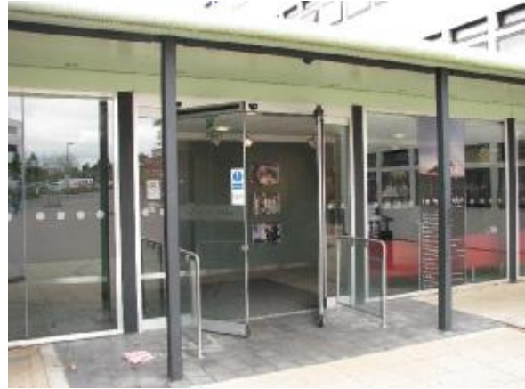
The foyer to the Nuffield theatre has automatic doors to both sides, with no obstruction to the air moving through one end of the foyer to the other.
