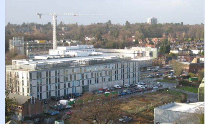
Site for the Life Sciences building before enabling works commenced in February 2008
