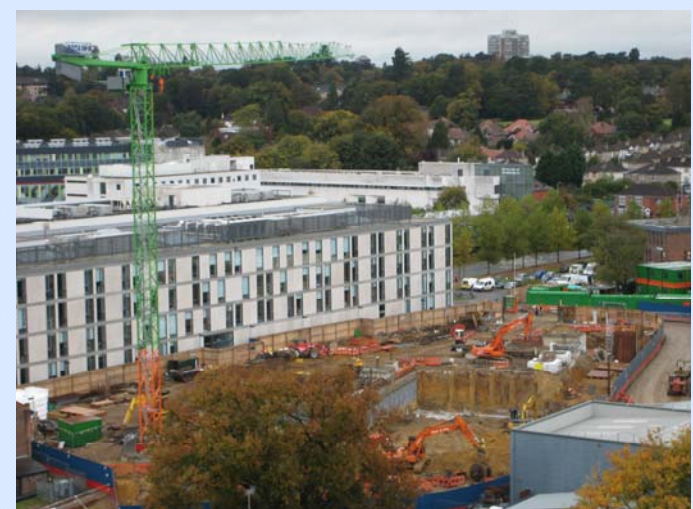
The first of the two tower cranes is installed on site
