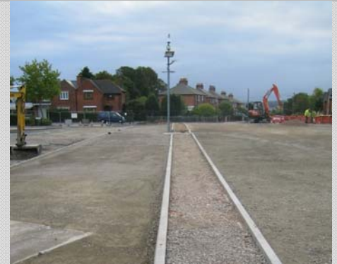
Resurfacing the Broadlands car park.
