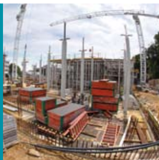
Construction work progresses on the new Mountbatten Complex
