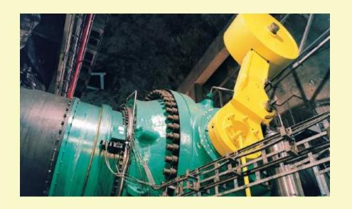
taps we call main inlet valves. Each valve can open in 5 seconds and allow 75.000 litres of water to pass through it every second.
