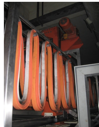
Figure 3 Flat form cables for the hoist
