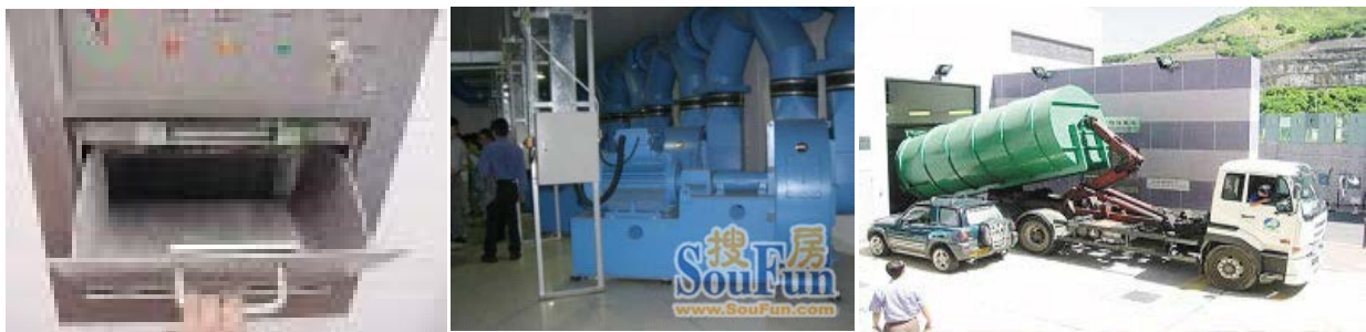
Figure 4.24: Pneumatic Waste Collection System In Tianjin Eco-City, taken from http://www.tianjinwe.com/tianjin/tjyw ; http://img.soufun.com/news/2011_07/29/news/1311929289172_000.png
