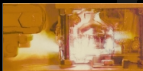
Figure 8: Arcing in a Miniature Circuit Breaker
