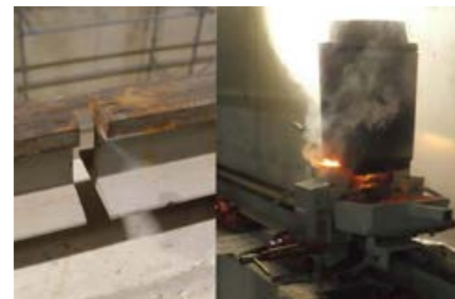
Fig. 6 Rail welding
